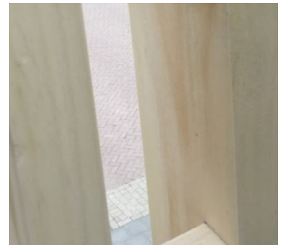
8.5 Reddish brown staining
